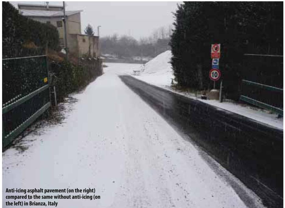
Anti-icing asphalt pavement (on the right) compared to the same without anti-icing (on the left) in Brianza, Italy
